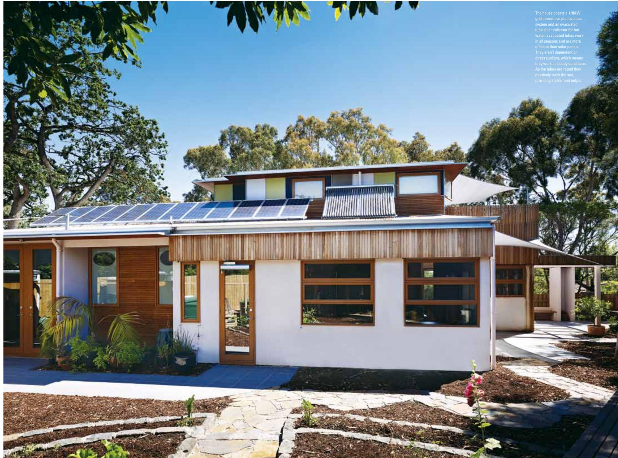
The house boasts a 1.98kW grid interactive photovoltaic system and an evacuated tube solar collector for hot water. Evacuated tubes work in all seasons and are more efficient than solar panels. They aren't dependent on direct sunlight, which means they work in cloudy conditions. As the tubes are round they passively track the sun, providing stable heat output.
